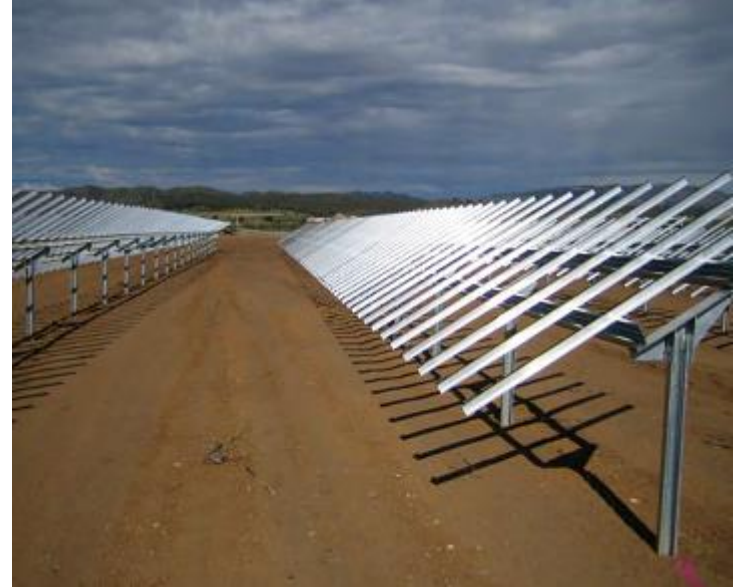
Static Pressure Piles
