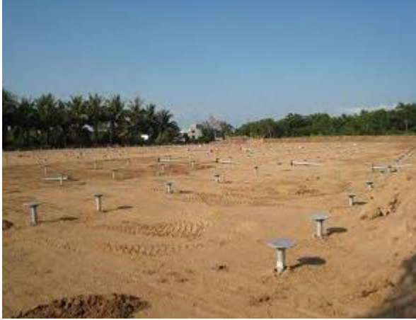
Screw drilling piles
